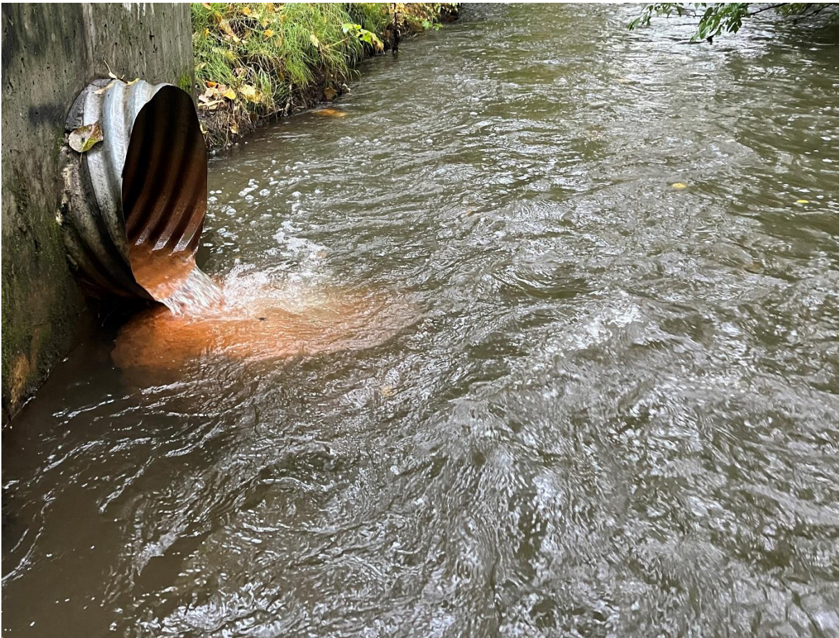
Photograph 8. Outfall SWM10 (525-2), Eagle Street at Chester Creek.
