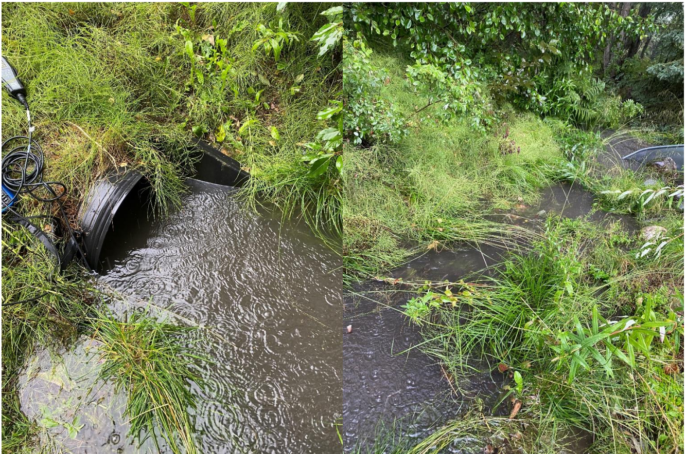
Photograph 2. Outfall SWM04 (1224-2), Fairweather Loop off Sylvan Drive.
