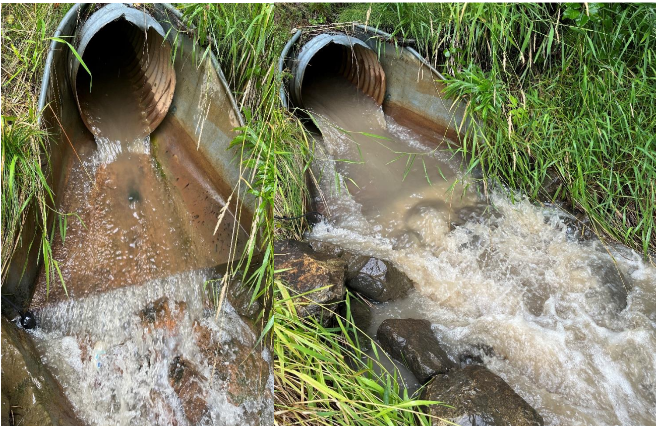
Photograph 10. Outfall SWM12 (1454-1), Lynwood Retention Basin.
