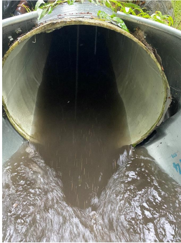
Photograph 1. Outfall SWM03 (1224-1), Fairweather Loop off Sylvan Drive.
